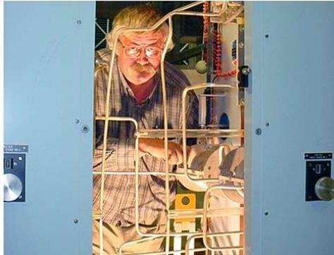
Older transmitters, such as the Continental 315R "Power Rock," employ older technology and are less sensitive to power problems. Newer Nautel transmitters are protected by three-phase power conditioners. Even with UPS and power conditioning, we occasionally see damage or failure, primarily for the computer-based gear that is becoming more common.
