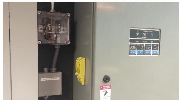
Figure 3 - The finished phase detector in operation.
