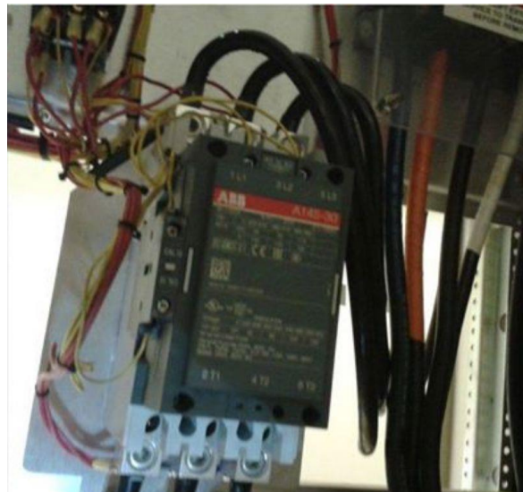
Figure 2 - The new contactor in place. Wonder how long it will last?
