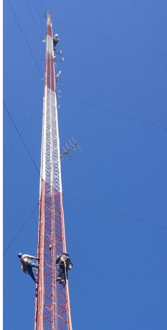
Figure 3 - Rigging to install a translator antenna for Guadalupe Radio.
