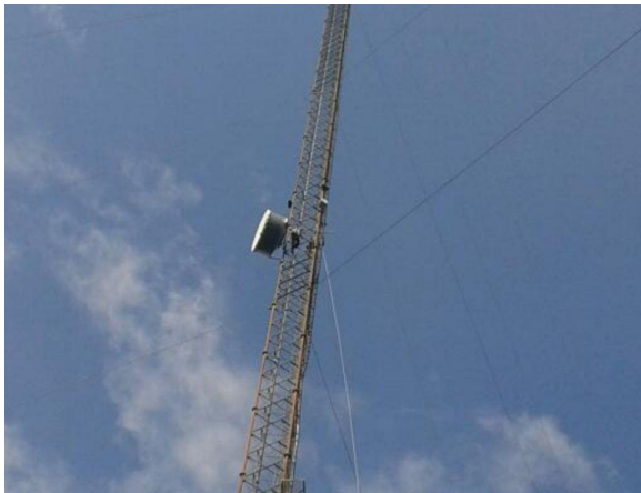
Figure 2 - Running the Fiber to the 8-foot dish at WYDE-FM.
