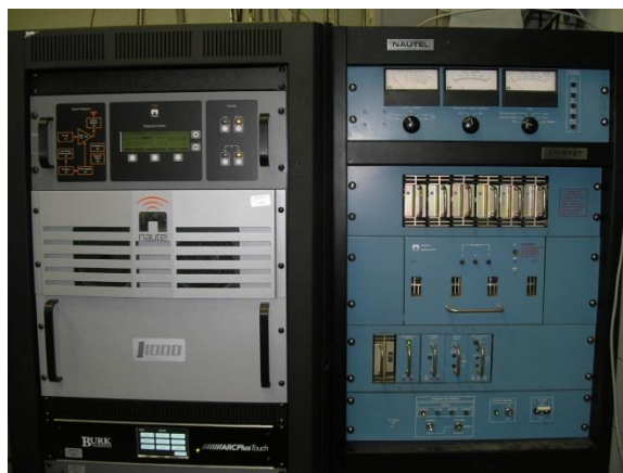
KNSN main (L) and aux (R) transmitters. Note the Burk ARC Plus Touch remote control below the main transmitter.
