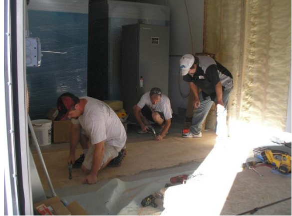
The ThermoBond crew installs the subfloor at the joint. Note the phasor cabinets and transfer switch in the east half of the building.
