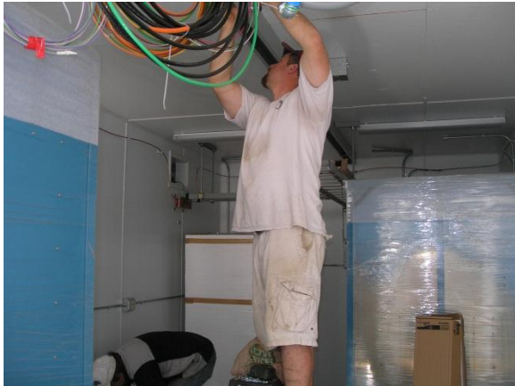
The ThermoBond crew installs the electrical duct to the west half.
