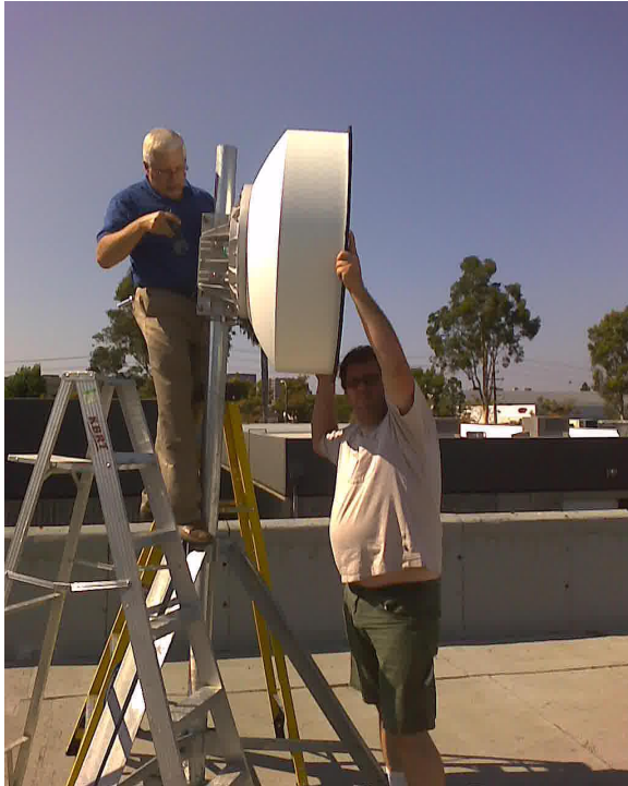
Bill Agresta holds the 11 GHz dish in place while I tighten the hardware. Note the heavy-duty tripod and mast.
