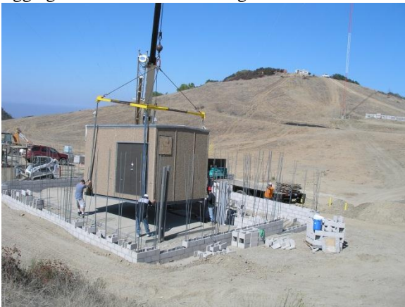
The east half of the building is placed on the slab.
