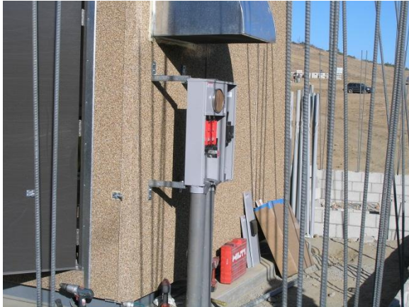
Service entrance and meter base installed and ready to go.
