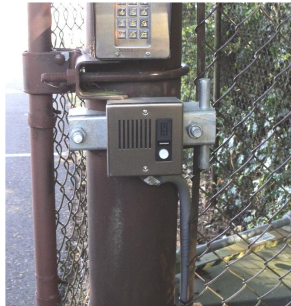
Completed call box at the gate.
