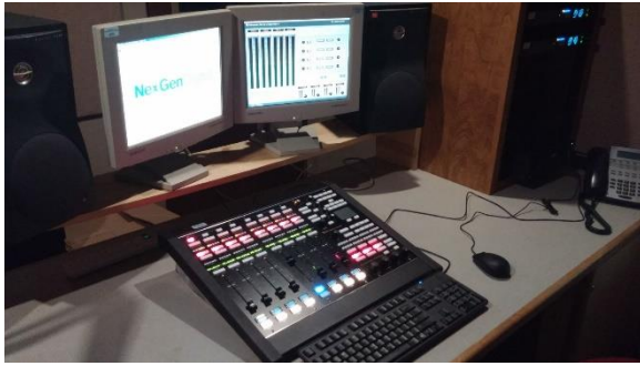
Figure 1 - Production 3 with the E6 Control Surface.
