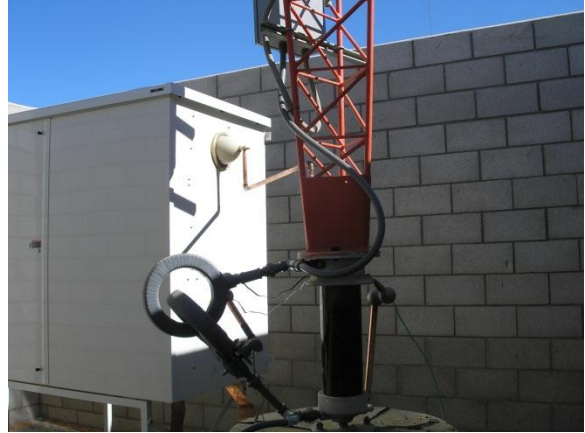
One of the tower bases with Austin transformer and feed tubing installed.
