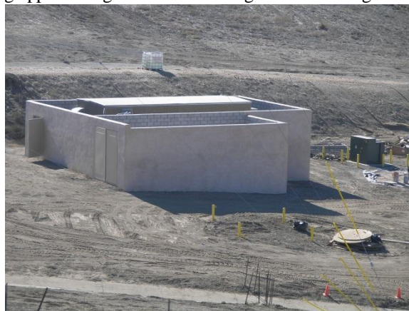
The KBRT Oak Flat transmitter building enclosed by stuccoed concrete block walls. The area beside the building is a stall for a portable generator.
