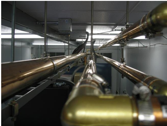
Interior transmission lines are all rigid, 3-1/8" and 1-5/8".
