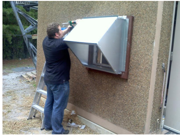
Figure 2 - Jimmy Parker caulking the weather hood for the new vent system
