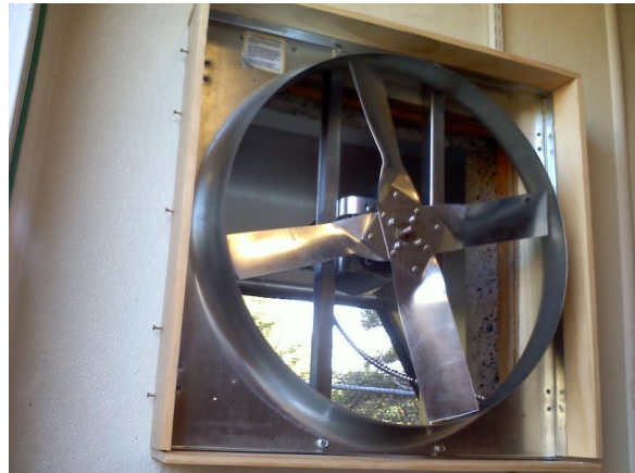
Figure 3 - Work in progress: the fan mounted into the existing hole
