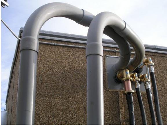
Cable entry to the transmitter building.
