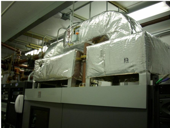
Exhaust ductwork for the new WDCX-FM NV-40 transmitter.
