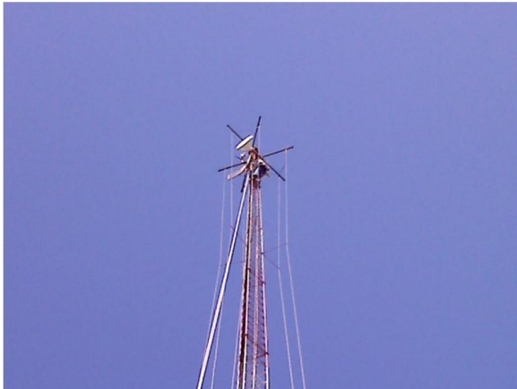
Figure 1 - Carefully mounting the Trango dish between the unipole lines at 1260.
