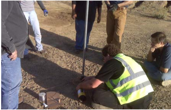
"Black Star Bill" solders ground radials to the ring at the antenna base.
