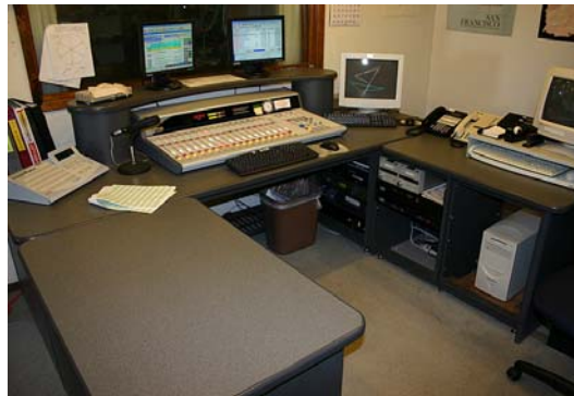
New KCBC Control Room Cabinets
