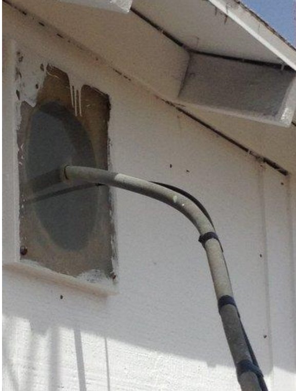
Air brake line was used as "conduit" to carry the fiber-optic from the control box on the tower through the doghouse insulator.
