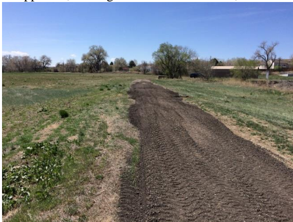
Recycled asphalt on part of the access road at the KLZ site.
