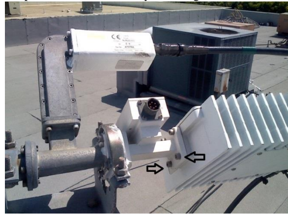
Figure 1 - New BUC on the KBRT uplink.
