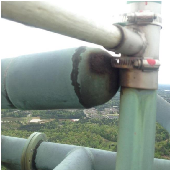
Figure 1 - A loose director contacting one of the bays was causing a bit of reflected power.
