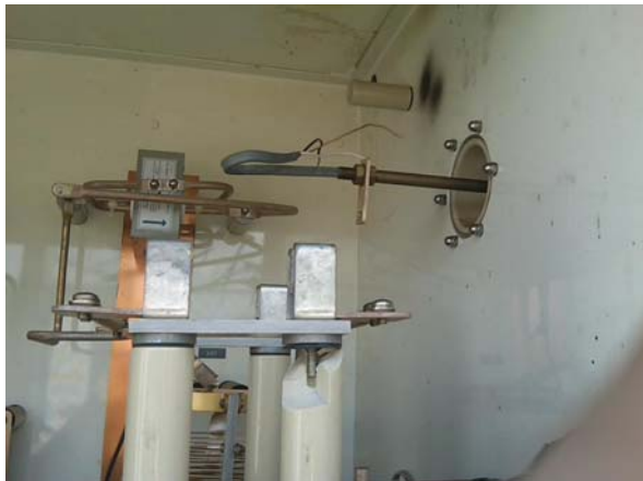
Preparing for Measurements at Tower 2
