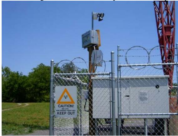
**Tower strobes are post-mounted inside the base fence**
