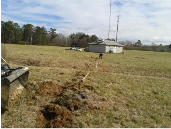
Jimmy Parker stuffing the new strap into the trench; Danny Dalton's backhoe is visible to the left.
