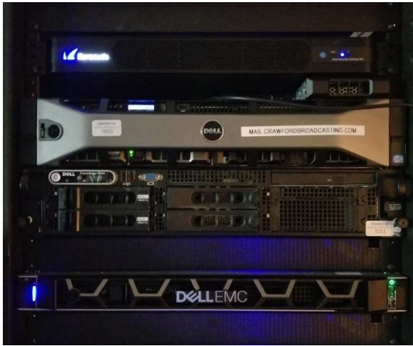
Figure 3 -- The new Dell firewall is at the bottom.
