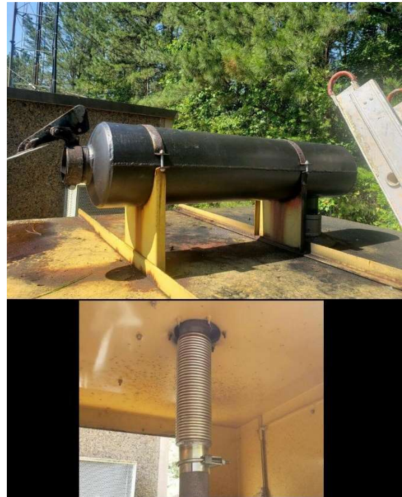
Figure 2 -- The new muffler and custom pipe work at WXJC-FM.
