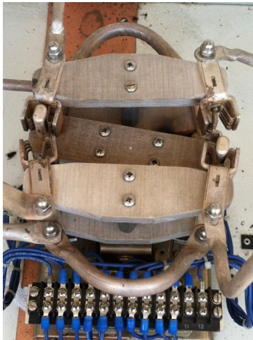
One of the RF contactors at KLTT.
