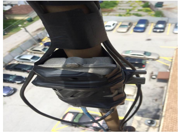
Figure 1 - We found the Ethernet surge suppressor attached to the tower with electrical tape. No ground wire was used.
