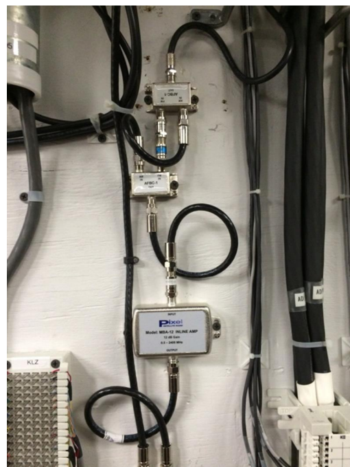
Figure 2 - Amplifier and pair of band splitters with a 20 dB attenuator between the FM ports.
