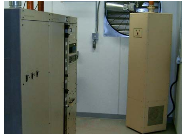
BE main transmitter and dummy load
