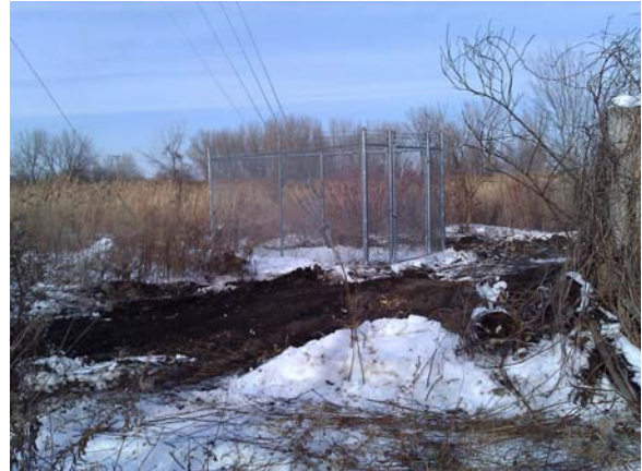
Clear paths to the guy anchors are needed for regular inspection and maintenance.
