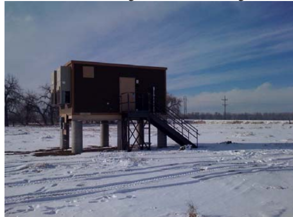
New KLVZ-D transmitter building with stairs
