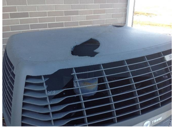
Ice damage to the A/C condenser unit at the WYCA tower site. The tower is several hundred feet east of this unit.
