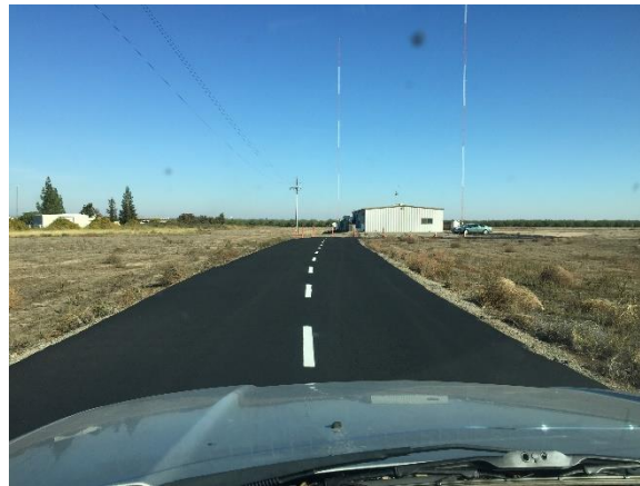
The resurfaced KCBC driveway. The white stripe is to help land planes...
