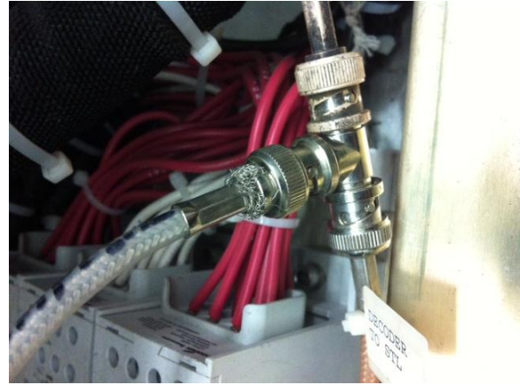
...but it isn't. Cold temperatures caused it to open up, killing baseband audio to the transmitter.
