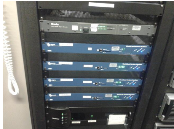
The APT Worldcast Horizon codecs carrying audio to the transmitter sites. The Moseley at the top is WDJC's 950MHz backup link, and the Intraplex at the bottom is for WYDE FM.
