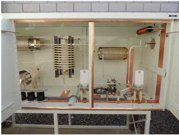
The tower #2 ATU - the 40-amp coil mounted vertically just left of center is the "resonating" shunt coil that we had to finesse to get things to work at that tower.
