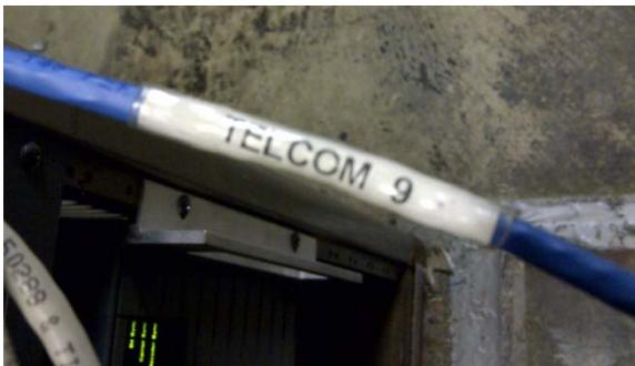
production sides. We tackled the symptoms as they popped up to ensure everything kept moving along while looking for the root cause of these issues. We again took a closer look at this area of the infrastructure and made some changes to the Firebox hardware firewall and to the wireless router. What further hindered us was the lack of proper labeling and tracking in terms of where the Ethernet cables went. Out of approximately 20 cables, only five or so
