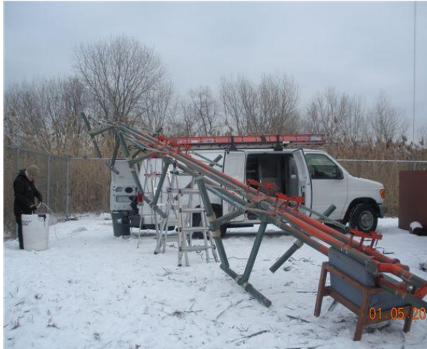
The WPWX antenna just as it reached the ground... total weight: 800 pounds!
