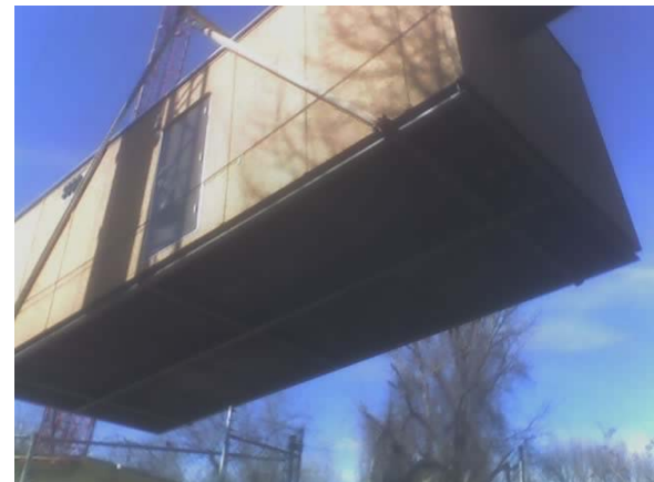
New WDJC-FM transmitter building being set into place
