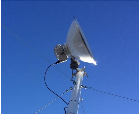
Figure 3 - The Dragonwave temporarily moved well above the heads of roofing crew.
