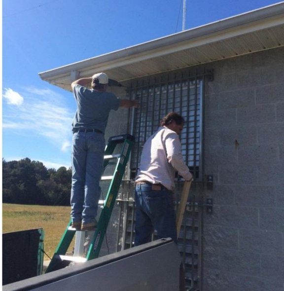
Figure 1 - Sunbelt Builders installing security bars at 850 AM.
