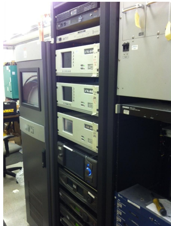
New NV5 transmitter and rack layout (WorldCast NextGen codecs are visible at the lower right).
