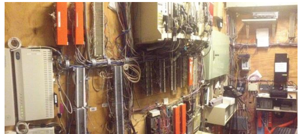
WMUZ telco room -- not a square foot available for the new phone system
