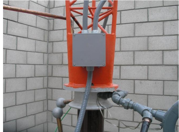
This PVC junction box routes the power wires and f/o cable from the microwave radio on tower 1 to conduits to the tower light control box and the PVC (non-metallic) conduit to the ATU cabinet.
