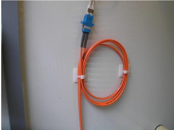
The fiber-optic cable from the microwave transceiver on the tower splices to the f/o cable from the building on the inside wall of the tower #1 ATU.
