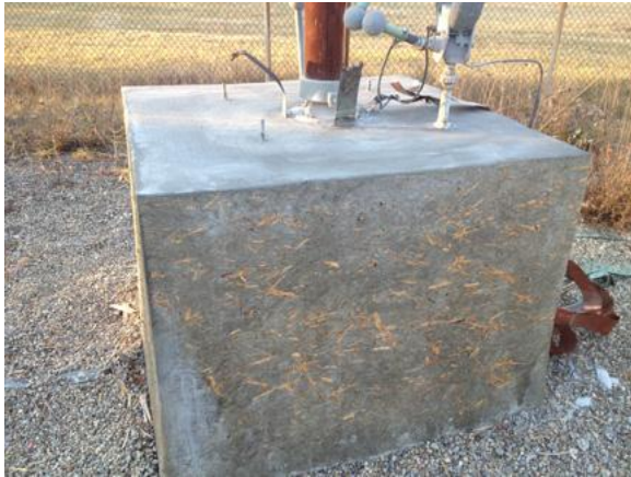
Finished recasting, before reattachment of ground straps.
