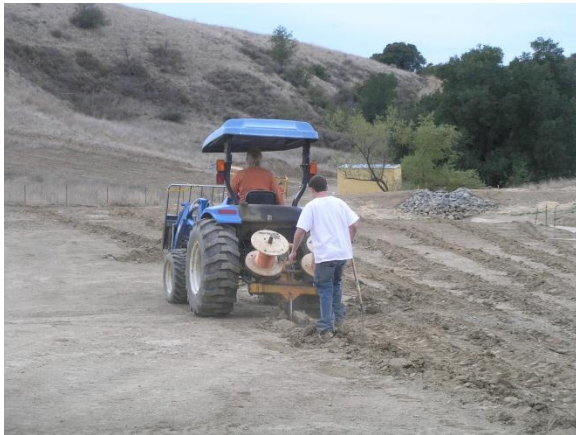
The crew from P&R Tower plows in radials.
