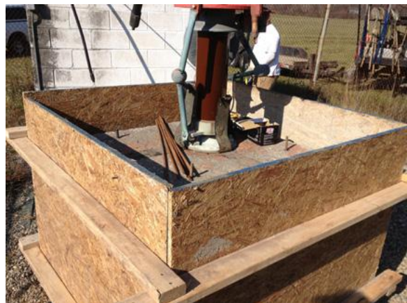
A form was constructed to hold the concrete in place until it cures.
