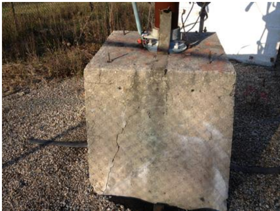
Cracked tower pier (Tower 4) WRDT-AM, before restoration
