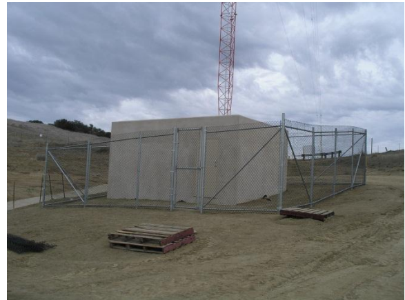
Tower base fences are complete. We used PVC-coated fence fabric to eliminate the contact burn hazard and the need to ground the fences.
