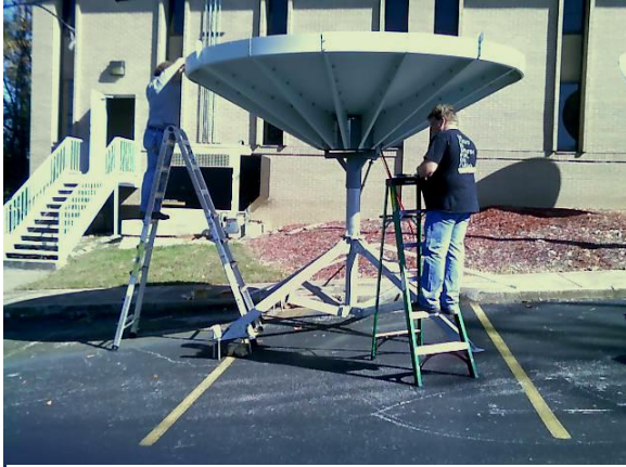
Todd Dixon and Jimmy Parker assemble the 3.8-meter Patriot antenna
