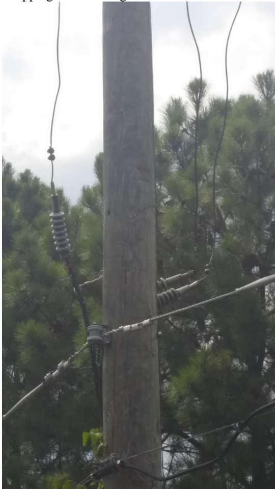
Not a great picture, but look at the insulators on the right. This is after the tech spread them.
