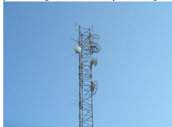
The 80-foot Pirod free-standing STL tower at the studio. Note the static dissipaters on the top.
