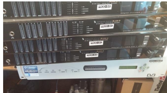
Figure 2 - Getting ready to install our Wheatstone blades.
