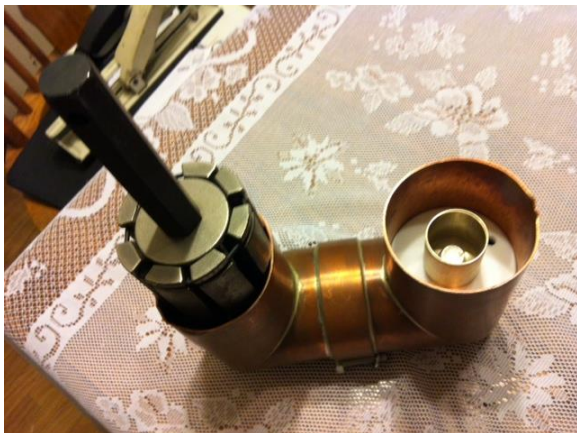
Figure 5 - Restoring the U-patch to round
