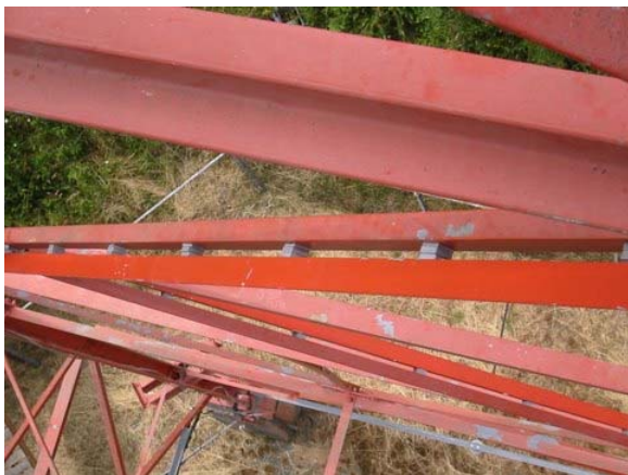
The new tower diagonals are clearly visible next to the old.
