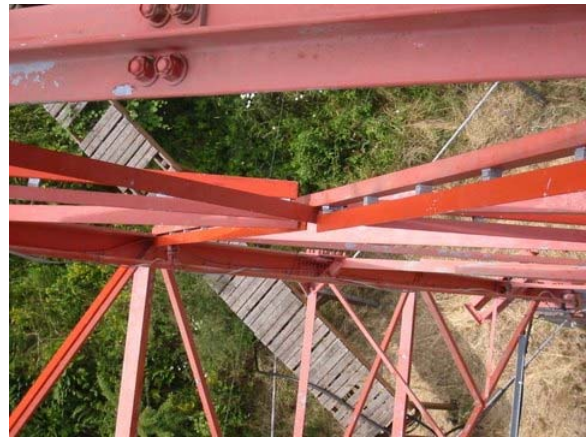
The new tower diagonals are clearly visible next to the old.
