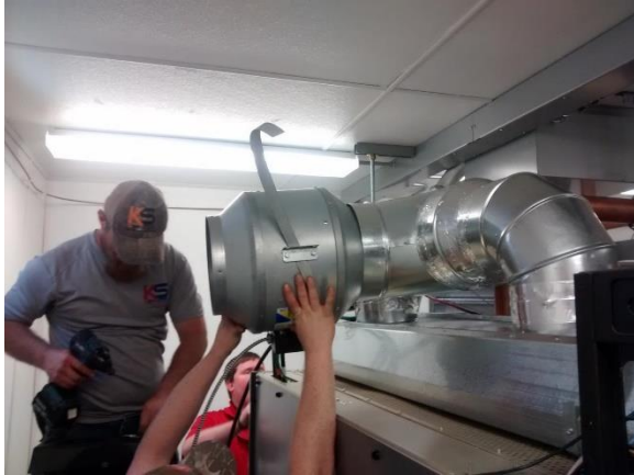
Figure 3 - New vent hood and fan being installed over WDJC's GV40.
