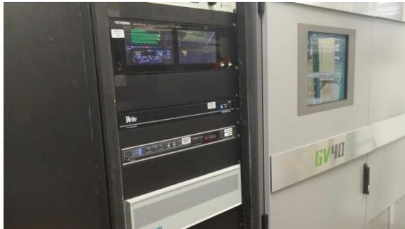
**Figure 1 - The new GV40 being driven with AES from the Vorsis AirAura3 processor.**
