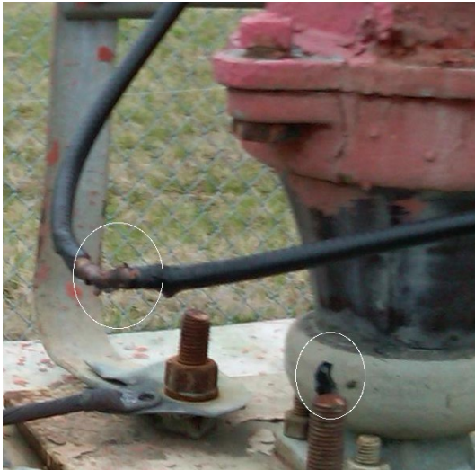
Figure 3 – Sample line pushed into the base by a severe storm
