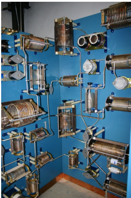
The new night phasor was built "Canadian Style" on laser-cut open panels
