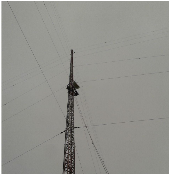
Figure 1 - Mounting the 11 GHz dish at 100 feet on tower #2
