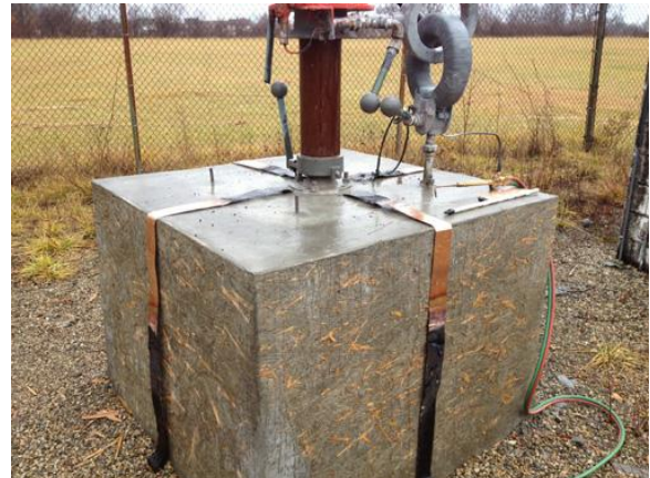
Completed ground strapping, tar application pending.
