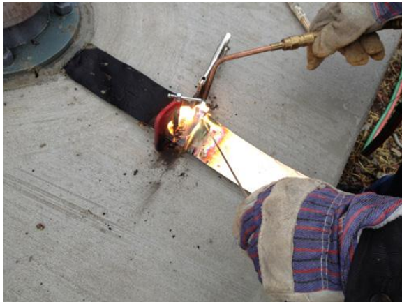
Brazing the new strap to the stubs of the old.
