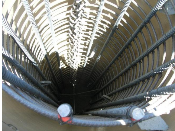
The rebar cage at tower #4 is in the hole and ready for concrete
