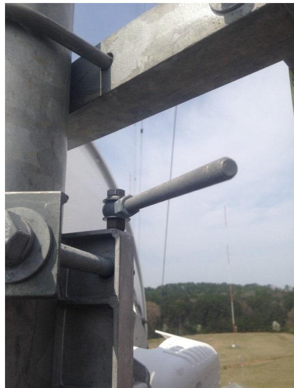
Figure 3 - The AZ adjust at Tarrant swings gently (and uselessly) in the breeze
