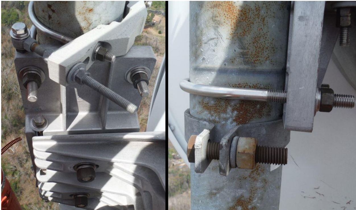
Figure 2 - Left: the AZ adjust incorrectly placed on top. Right: a cheesy, thin clamp supports the entire mount at the bottom
