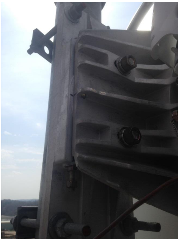
Figure 4 - At Tarrant, the factory-supplied hardware was replaced with flat clamps and all-thread
