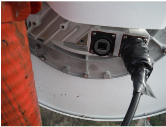
Figure 1 - Note the unused data port was left uncapped, and note the missing ground wire at the unpainted connection point to the left of the unused port.
